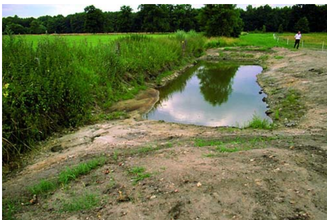
Fig. 9: View in flow direction of the „Sediment trap Bargfeld“ in summer of 1999 about one year after completion and after the first time of excavation. In front of the left side the mouth of the drainage ditch can be seen. At the far end on the left of the sediment trap the drainage ditch continues its flow through dense vegetation.
